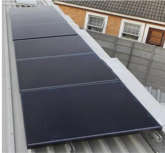
By connecting it in PARALLEL the system voltage remains at 87,5V, while the power still adds up to the total of 1,02 kW. This means a maximum current of 11,7A.
